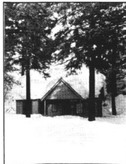
High Bridge Guard Station
