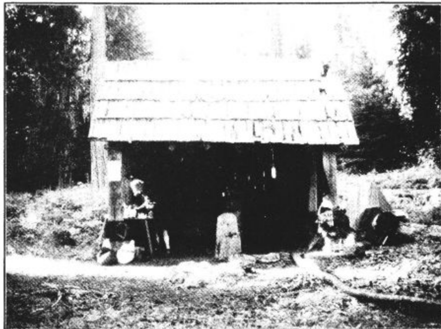
Cripple Creek shelter.
